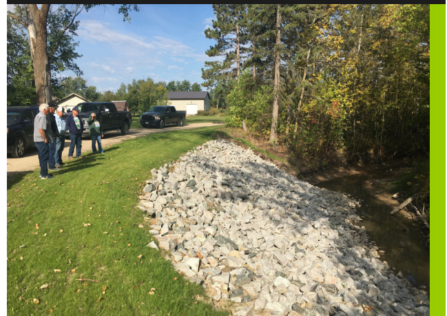
Fast Streambank Restoration Site The project used rip-rap armoring.
