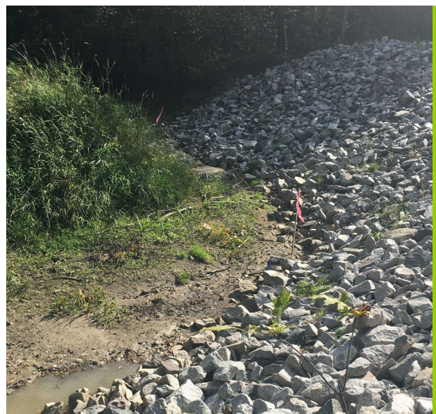
Phillipe Streambank Restoration Site The project utilized rip-rap armoring.
