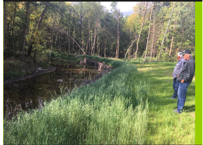
Ulwelling Streambank Restoration Site The project utilized natural armoring / anchoring materials such as root wads, vegetation installation, and strategic placement of on-site fallen trees.
